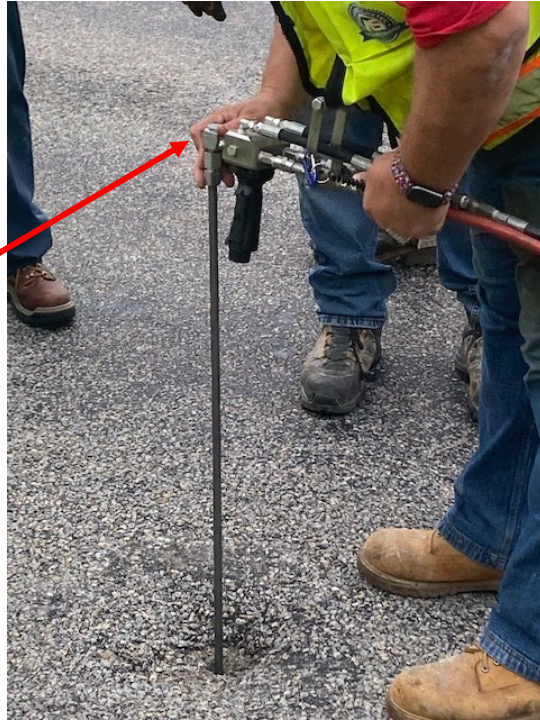
MixMaster deep injection attachment
