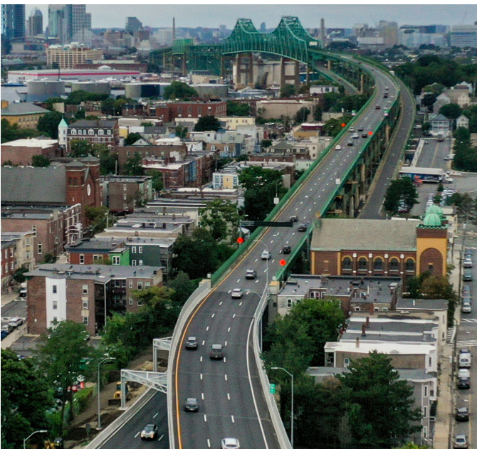
Newly replaced deck, new pavement markings, and installed snow fence. Photo: August 2021
