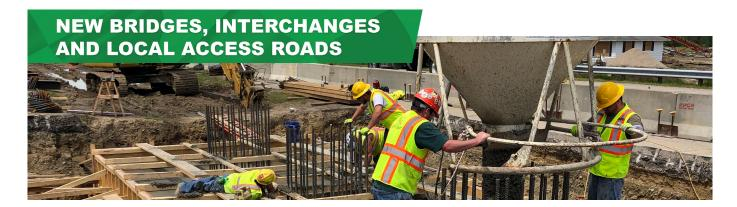
Crews are moving dirt in several areas to begin building new local access roads parallel to S.R. 37 that will connect with future overpasses and interchanges. Crews are driving steel pilings and pouring concrete footers for new bridges over S.R. 37 near Egbert Road, Henderson Ford Road, Perry Road and Waverly Road. Drivers can expect lane closures in the area.
