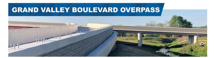
The Grand Valley Boulevard overpass is nearing completion and will provide a new east-west connector for drivers and pedestrians. Concrete forms and wooden working platforms have been removed, revealing new concrete decking and railings.
