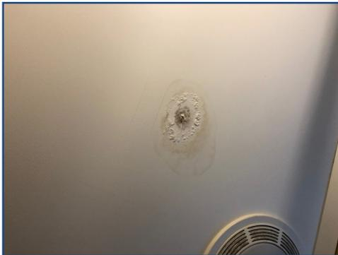
**Figure 2:** Water damage/possible mold.
