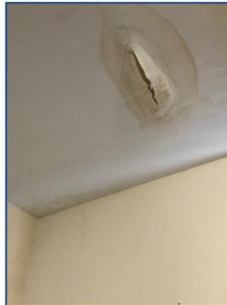
**Figure 3:** Water damage.
