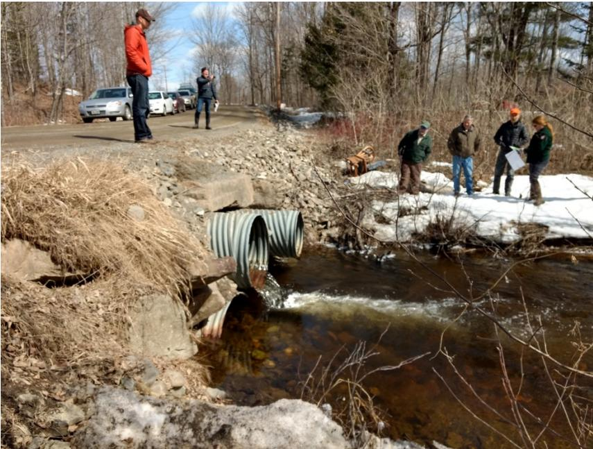
**Figure 6. Perched and undersized culverts proposed for replacement at the crossing of Bacon Rd. over an unnamed tributary of Crooked Brook**
