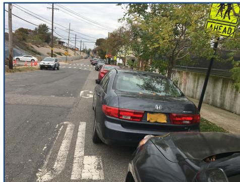
**Image 2** (facing north): Damaged “School Crossing” pavement marking on the southern leg of Montauk Street
