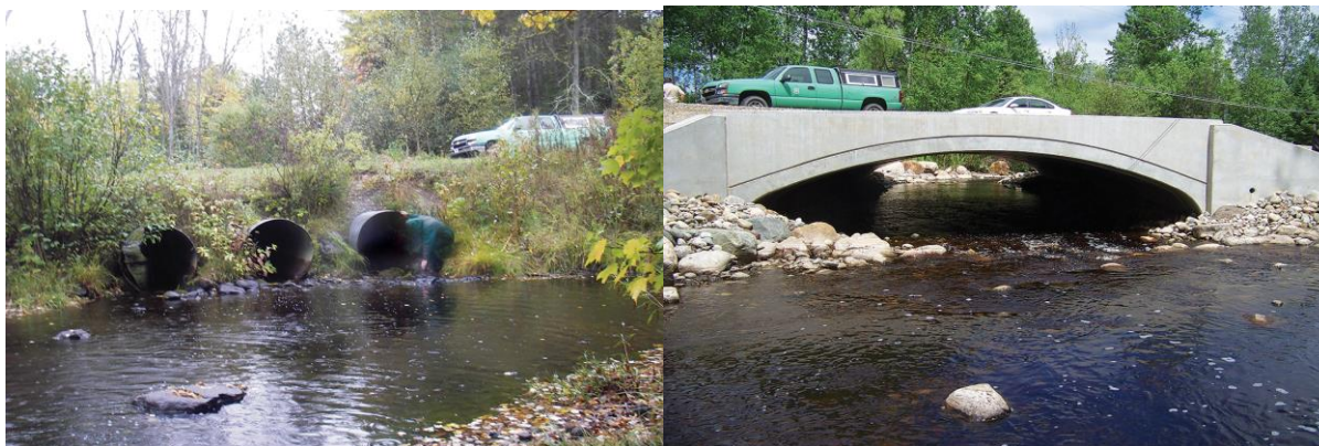
Figure 3.6. Replacement of perched culverts. The “perched” culverts in the figure on the left prevent upstream fish movement, whereas fish can move through the natural stream channel bottom under the concrete arch in the figure on the right.
