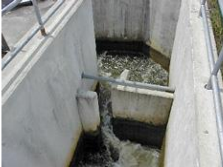
Figure 3.7. Image of a vertical slot fishway.
