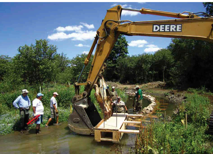
Installing lunker structures
