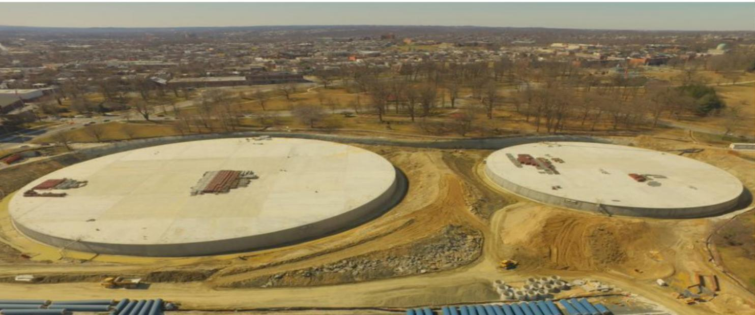
The City's iconic Druid Lake holds filtered and treated water that is ready to be delivered to consumers. At this site, two massive underground tanks are being built to protect this drinking water supply.
