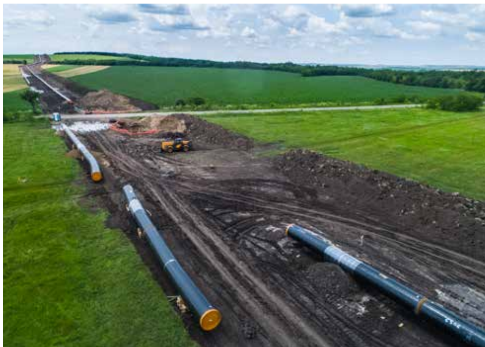
Aerial view of pipes at a construction site of a natural gas plant
