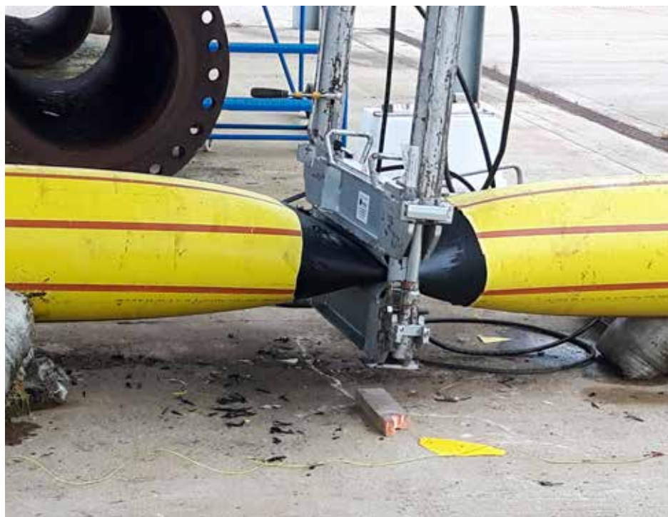
An example of a 'squeeze off' flow-stopping method on a polyethylene pipe
