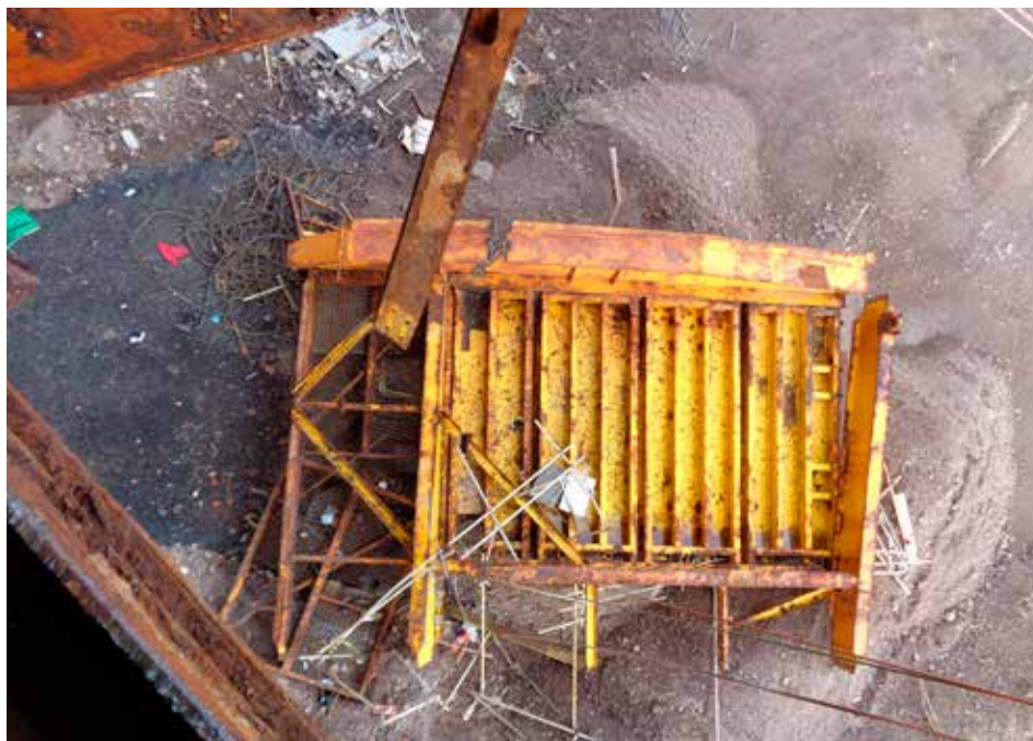
Collapsed platform seen from the main structure
