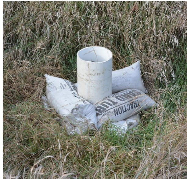
Figure 1: Block tile inlets if runoff conditions are present.
