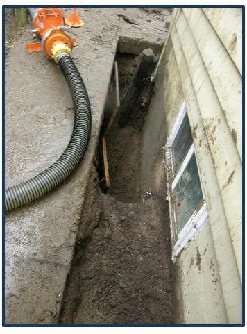
Incident scene showing the unprotected trench measuring 21 inches wide by 60 inches long and 7 feet deep that collapsed, burying the victim. This photo was taken after emergency responders removed the victim.
