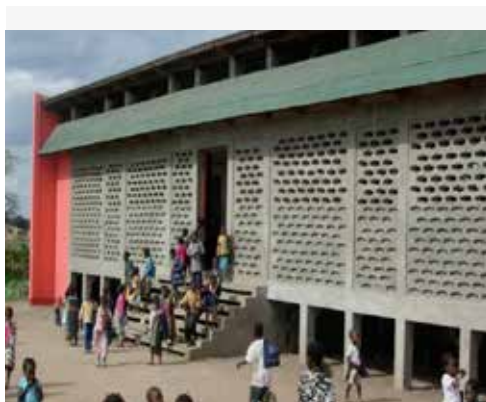
IMAGE 13 A, B. Infrastructure of education. Elevated school construction protects from flooding. Reinforced school roofs protect from cyclones.
