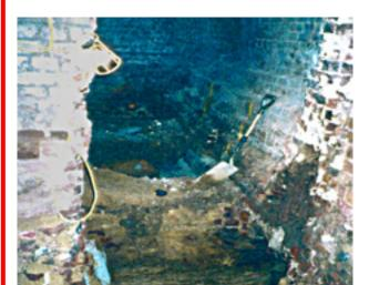
A large central mass of soil was left unsupported in this basement conversion. It collapsed on a worker, killing him.
